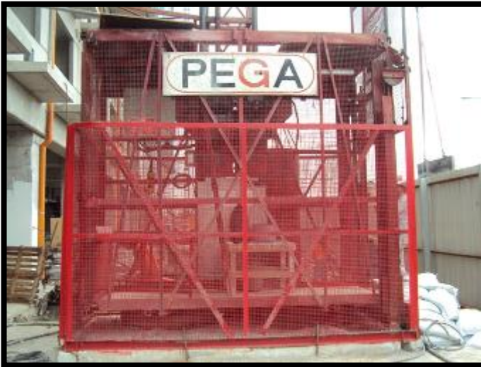
Inspection and Load Testing of Construction Elevator at Megawide Building Project
