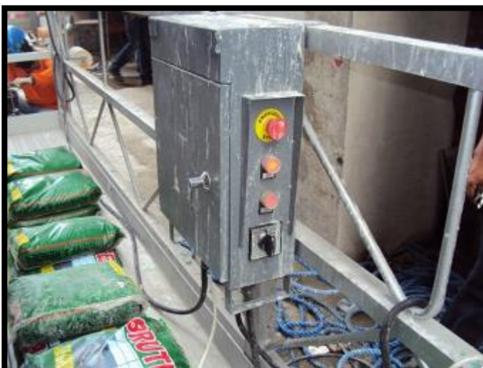
Inspection and Testing of Gondola Sea Residences Project
